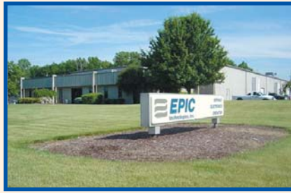
EPIC's headquarters in Rochester Hills, MI.
